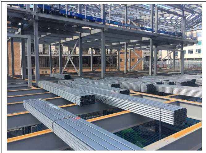
Netting and decking commenced to Zone 4.
