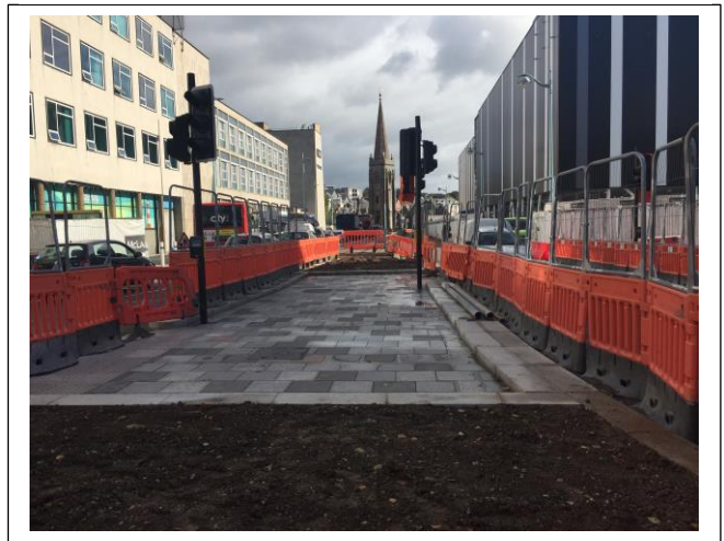
Paving and landscaping completed to St. Andrews roundabout.
