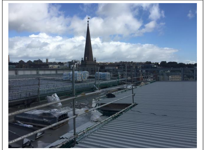
Roof works ongoing to Zone 3.
